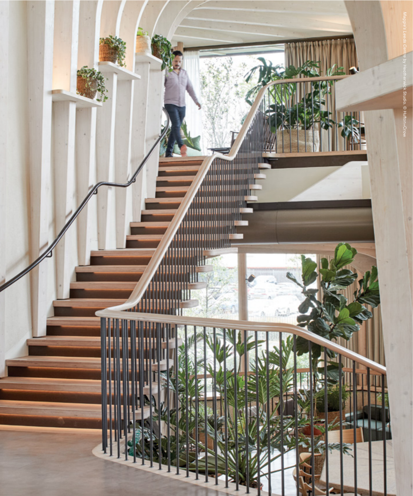
Continuous handrail from corridor to staircase, with rounded corners for a seamless connection.
