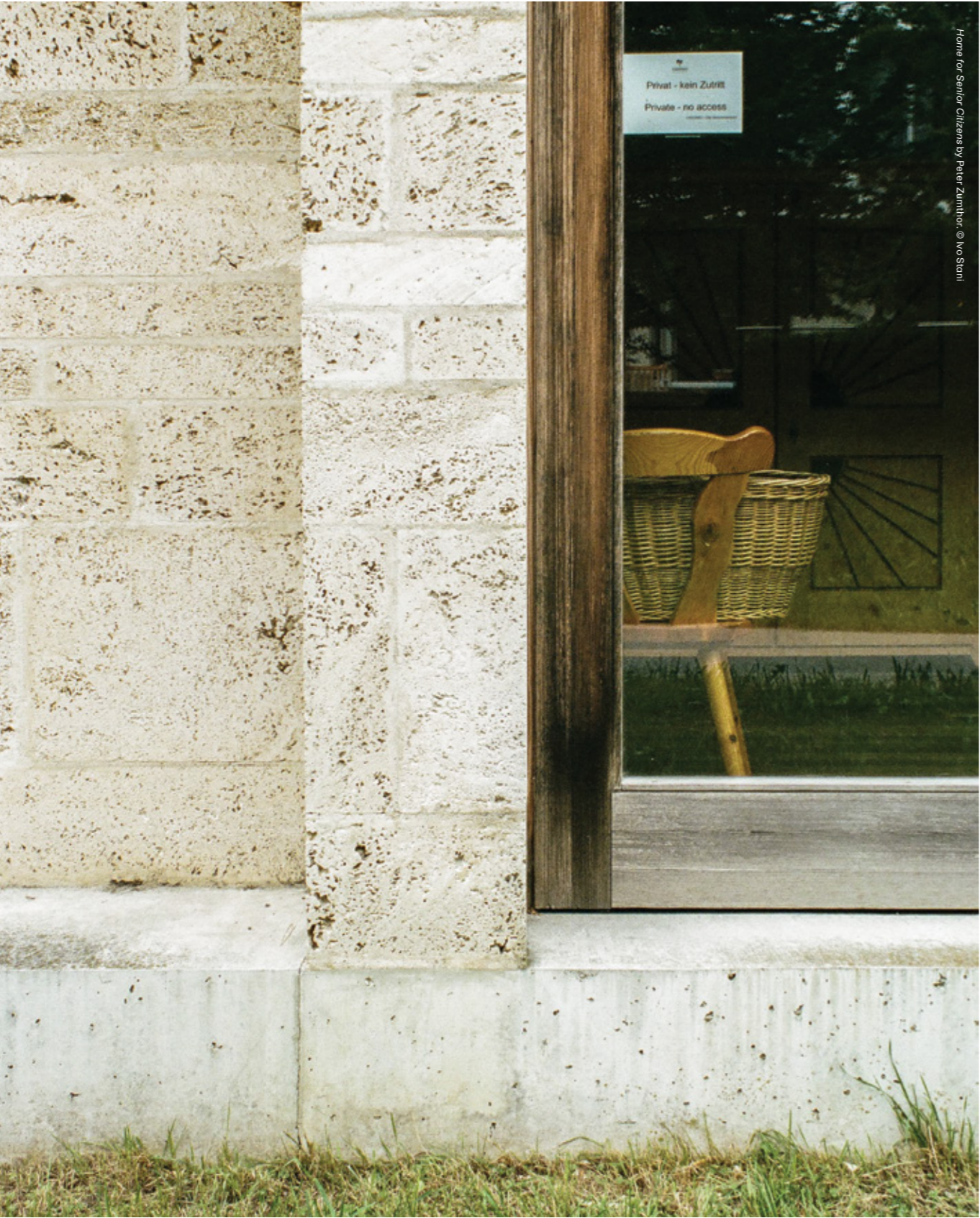
The use of materials like exposed concrete, tufa and larchwood creates a rural atmosphere in a suburban setting, inviting both new and long-term residents to feel at home. The choice is reinforced by clear construction details, resulting in a work of art that reflects familiar local elements.
