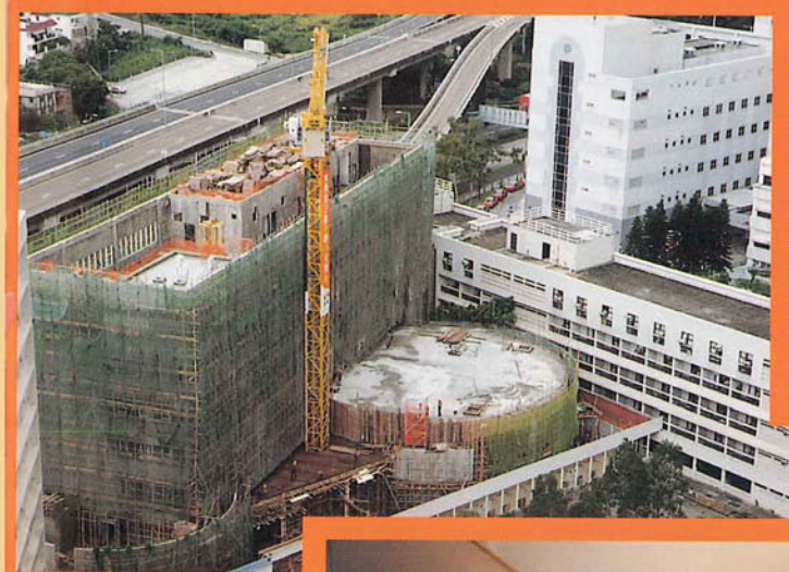
School of Public Health under construction
