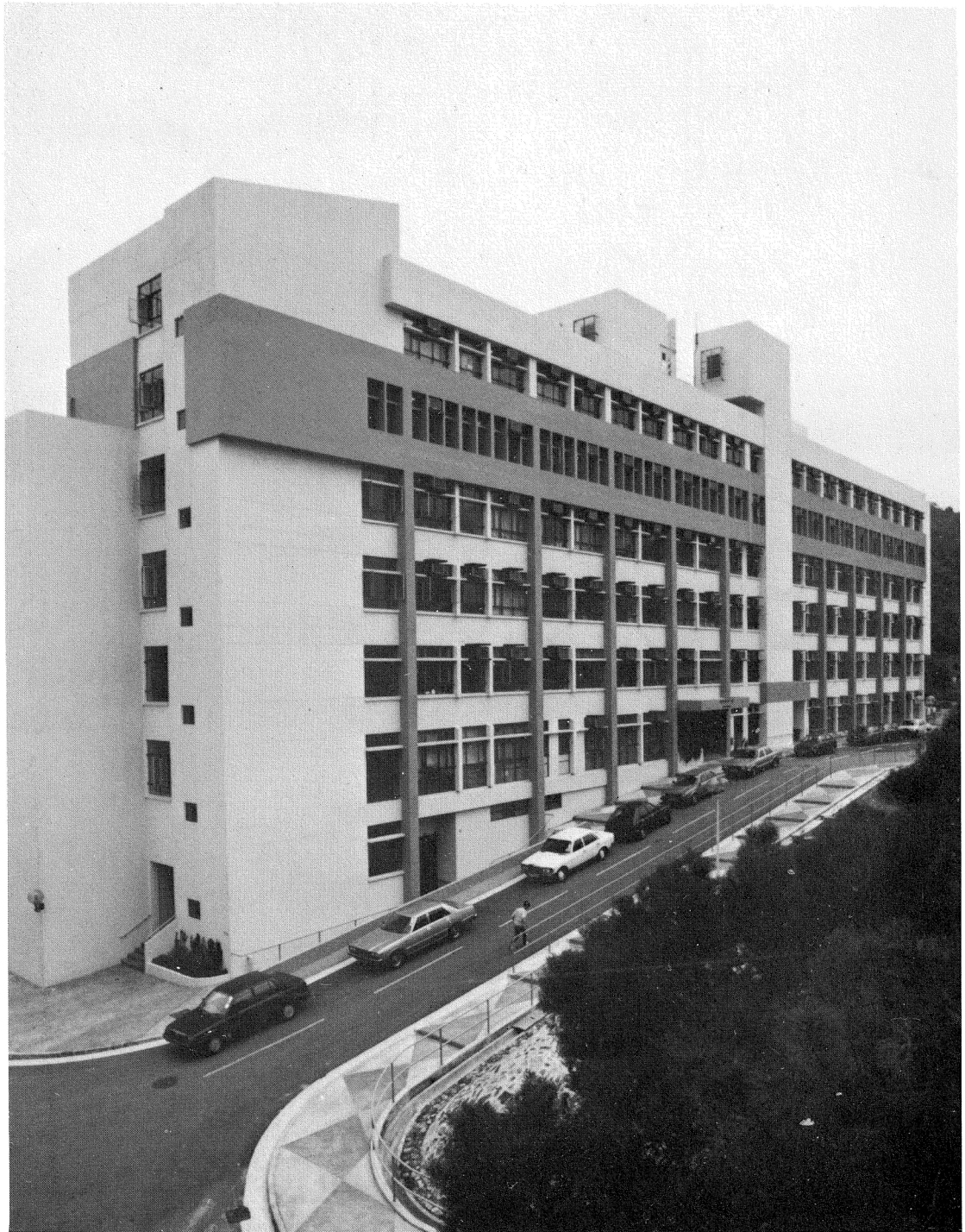
Fung King Hey Building
