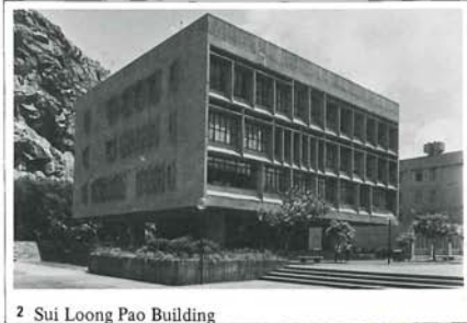
2 Sui Loong Pao Building
