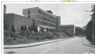
10 University Administration Building
