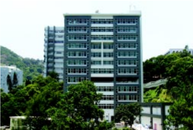
William M.W. Mong Engineering Building
