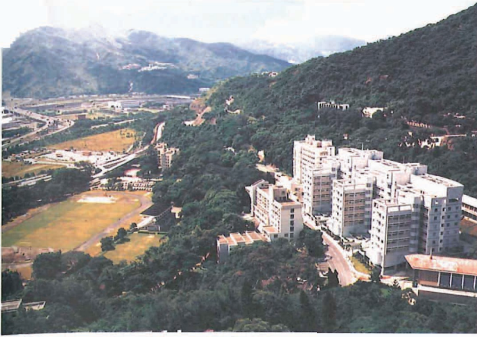
The teaching and administration blocks on Chung Chi campus
