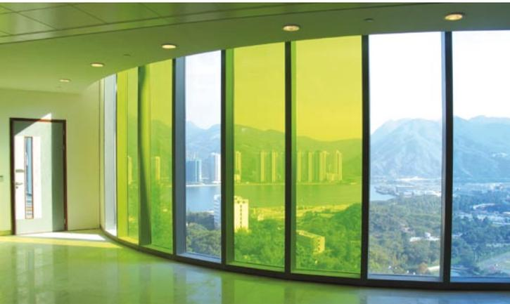
Storey-high, insulated glass units on the southern façade of the Centralized Labs
