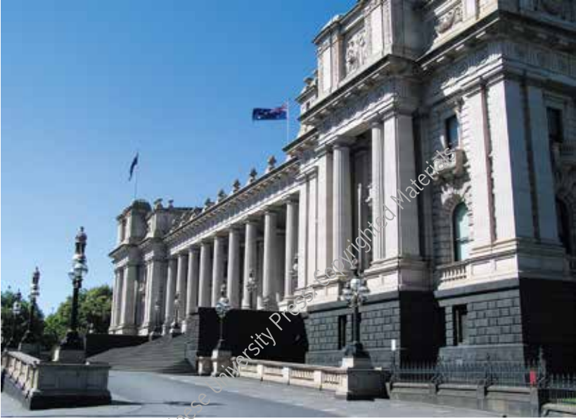
Figure 2.1 Victoria State Parliament Building in Melbourne 9
