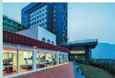
Full Sea View Gymnasium - The gymnasium overlooking Tolo Harbour is the perfect place to keep both body and mind fit.
