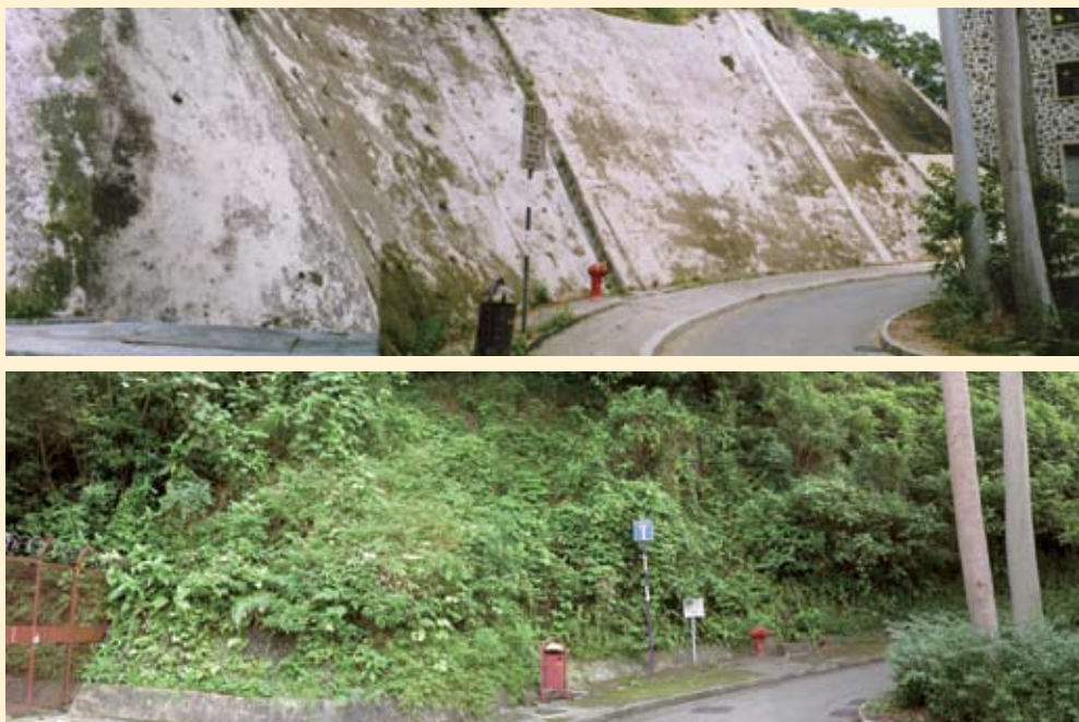
九十年代在崇基職員宿舍附近蓋滿灰泥護面的斜坡（上圖）；同一斜坡的現貌（下圖）。 Before: a slope covered with chunam plaster near Chung Chi staff quarters in the 1990s (top) After: the same slope now (above)
