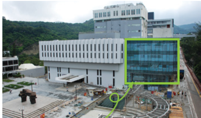
Library extension near completion
