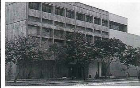
John Fulton Centre Usage: staff/student amenities Date of completion: December 1988 Funding source: Hong Kong Government
