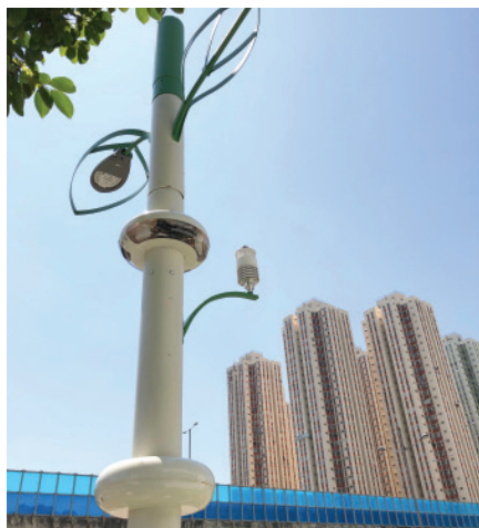
Figure 3. A smart lamppost on Shing Kai Road.
