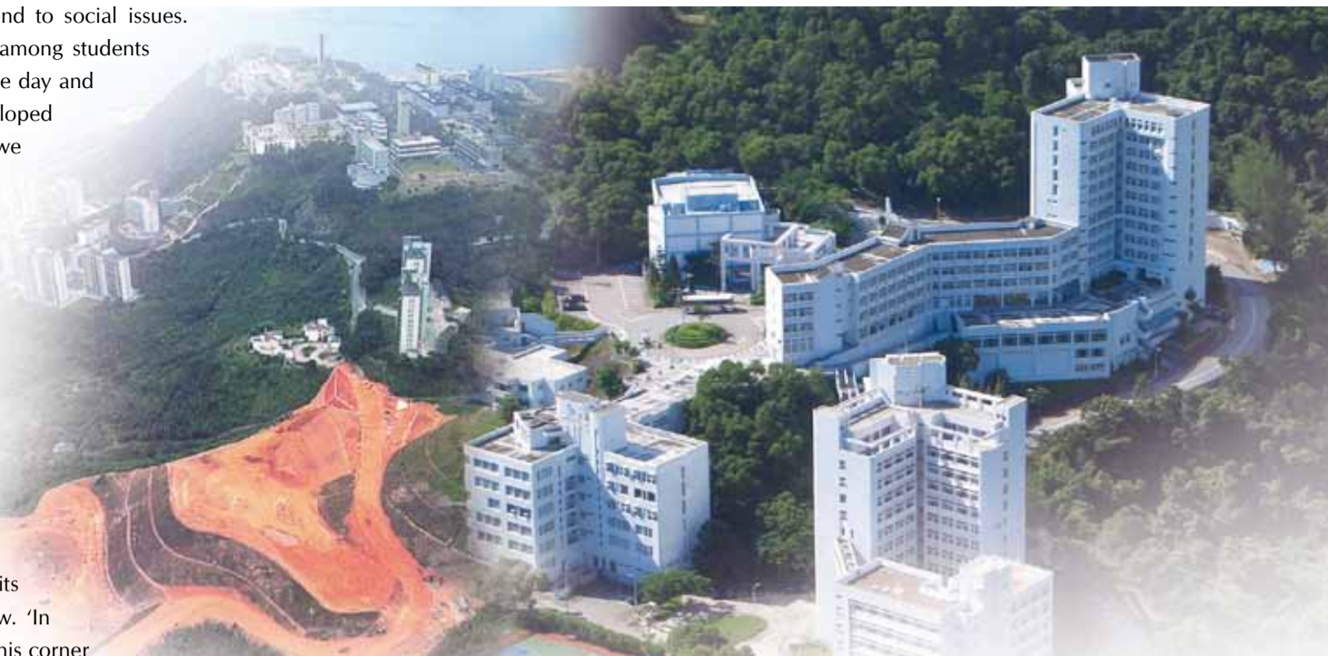
逸夫書院於1986年動工興建(左)發展至今(右)已具規模 Shaw College under construction in 1986 (left) versus the developed campus (right)
