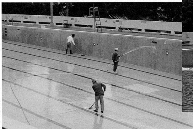
The sides and bottom of the pool are given a good scrub each year and missing tiles are replaced.
