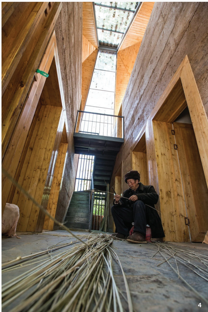
4 一專一村團隊為農宅設計了採光通風良好、舒適美觀的半室外中庭空間。 The semi-outdoor atrium built by the 1U1V team provides a comfortable and artistic living environment for the elderly villagers.
