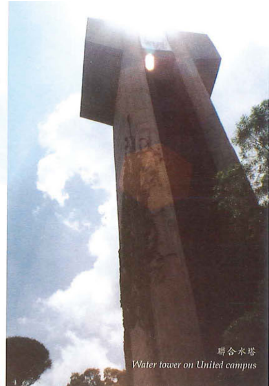
新亞水塔 Water tower on New Asia campus
