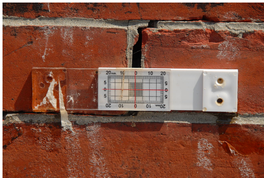
Ex: mechanical strain gauge used to measure the growth of a crack in a masonry foundation.
