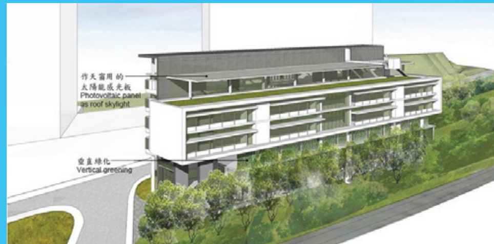
Solar panels and roof greening at the proposed Integrated Teaching Buildings 擬建綜合教學大樓的太陽能板和綠化天台
