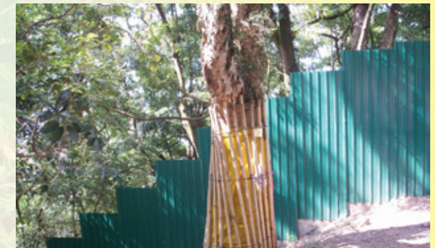
Protection of tree trunk from physical damage in a construction site
