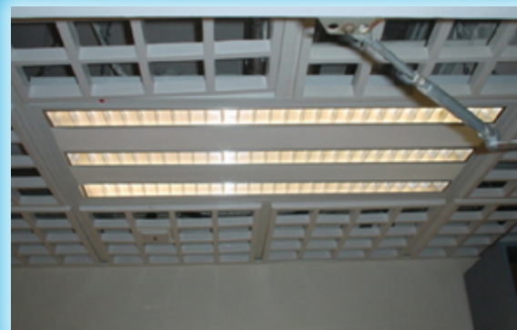
T4 Light retrofit project
