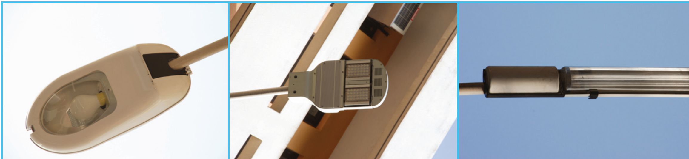
Lamp testing of electrodeless induction lamp, LED lamp & SOX lamp.
