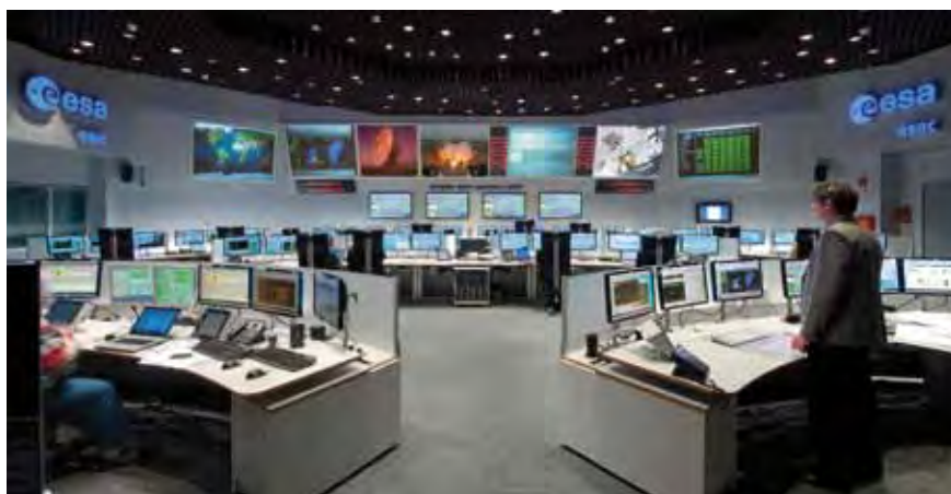
Figure 7.1. The main Flight Operations Control Room at ESOC, Darmstadt, Germany.
