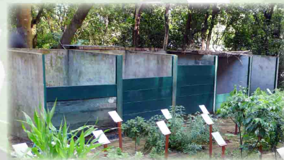
6. 堆肥槽 Dunghill Storage Hut
