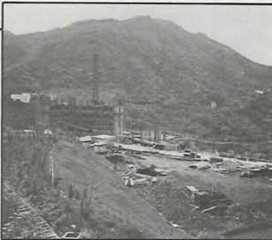
College buildings under construction
