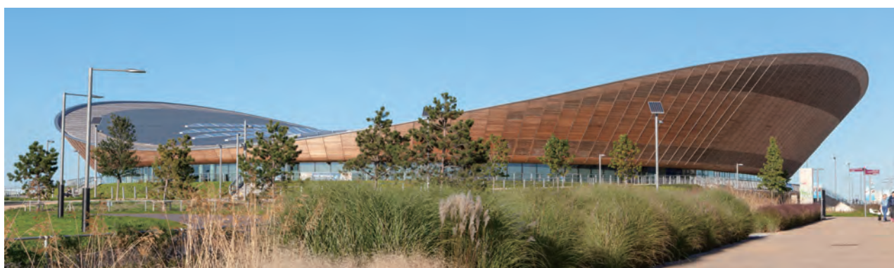
▲ 位於倫敦奧林匹克公園的室內自行車館，也是採用「雙曲拋物面」的幾何設計 The velodrome cycling arena located in the London Olympic Park also adopts 'hyperbolic paraboloid' in its design
