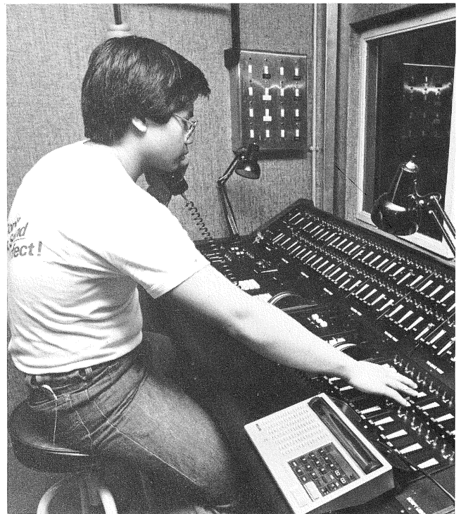
Lighting console in control room and intercom telephone
