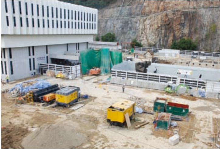
大學圖書館擴建工程 Construction of University Library Extension
