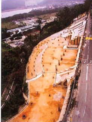
Aerial view of the building site in March 1998
