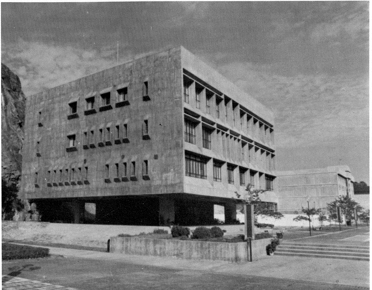
Sui-Loong Pao Building, which accommodates the Graduate School and various research units
