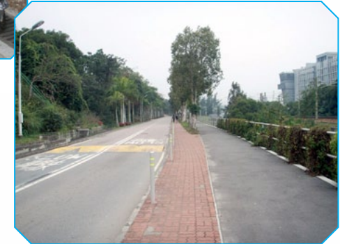
Cycling track between MTR station and Area 39
