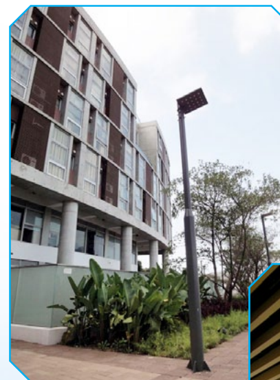
LED street lighting
