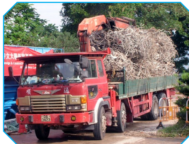
Metal wastes are sorted on site and sold to collector for recycling
