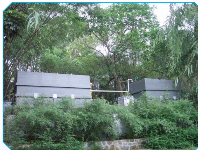
Construction of water treatment plant
