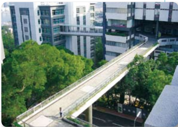
●● Bridge links between Engineering Buildings ●● 連接工程大樓的天橋
