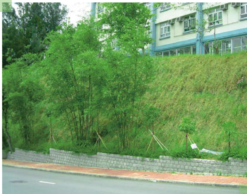
▲ A steep slope was made more gentle and fixed by soil nails, hydro-seeded and covered with an erosion control mat. 陡峭的斜坡經過處理，減低斜度，並安裝泥釘，以濕法噴播植草，再鋪上保護席。
