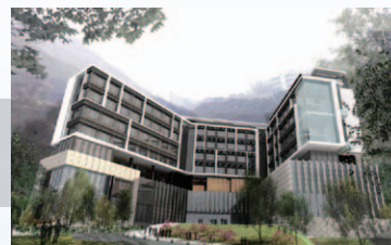
Façade of the College Campus
