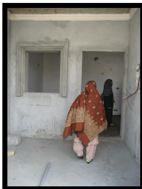
Figure 3: This is the actual house which Jannat bought. Her mother and sister are inspecting the place during the construction progress.
