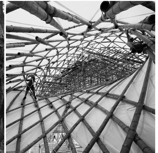
from left to right: g9 retaining wall; g10 zcb bamboo pavilion by kristof crolla.
