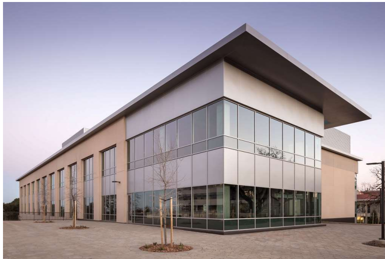
SLAC's Arrillaga Science Center – Nanofabrication facility , 2019
