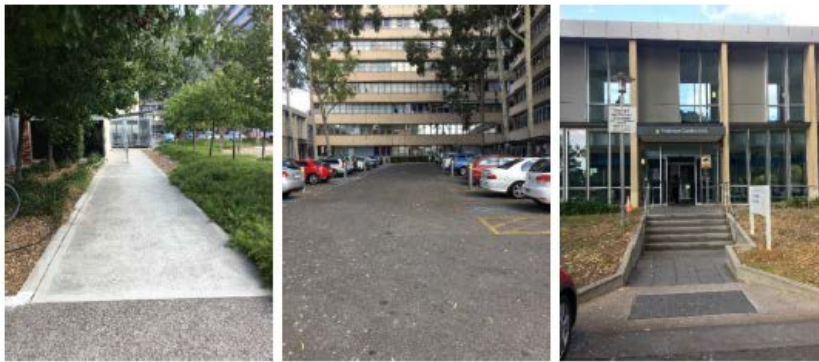
Figure 7. Obstruction in the middle of a footpath (left); no dedicated footpath to carpark (centre); no ramp to a building (right)
