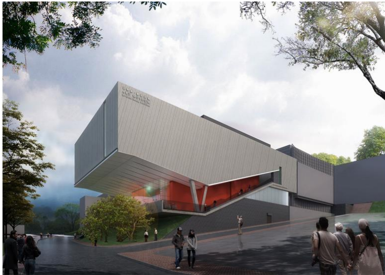
Art Museum of The Chinese University of Hong Kong – Lo Kwee Seong Pavilion under Construction
