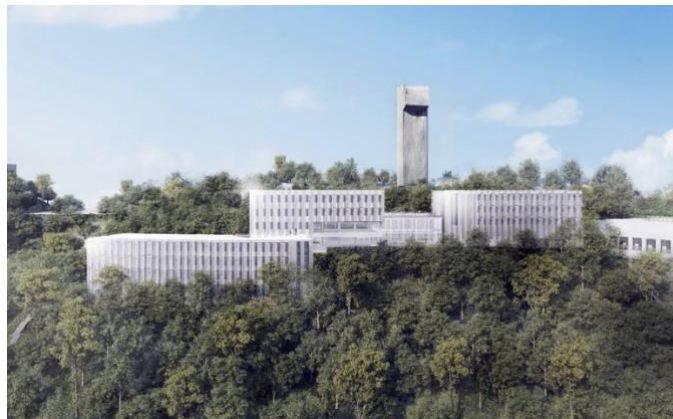
New Hostel under Development
