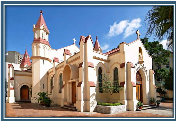
Photo: Rosary Church after renovation in 2003
