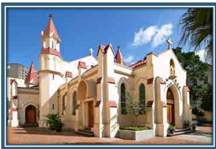
Photo: Rosary Church after renovation in 2003
