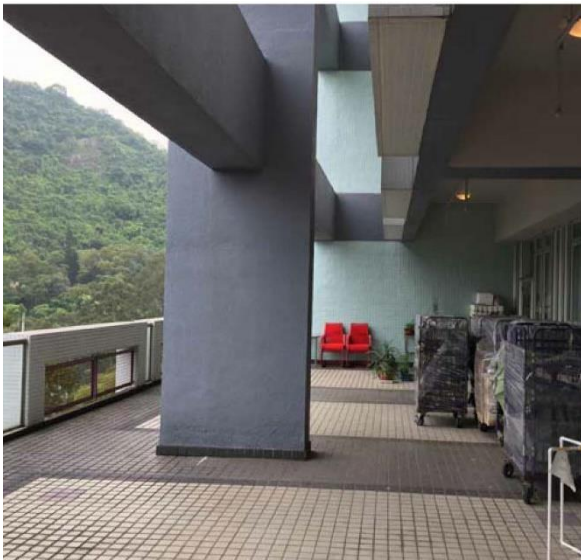
2/F Flat Roof (before renovation)
