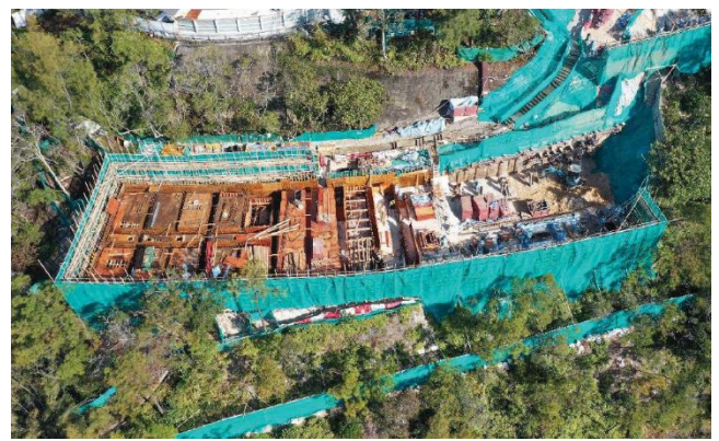
Pile Cap Preparation Works at Lower Platform in Progress – Block 1
