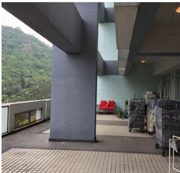
2/F Flat Roof (before renovation)
