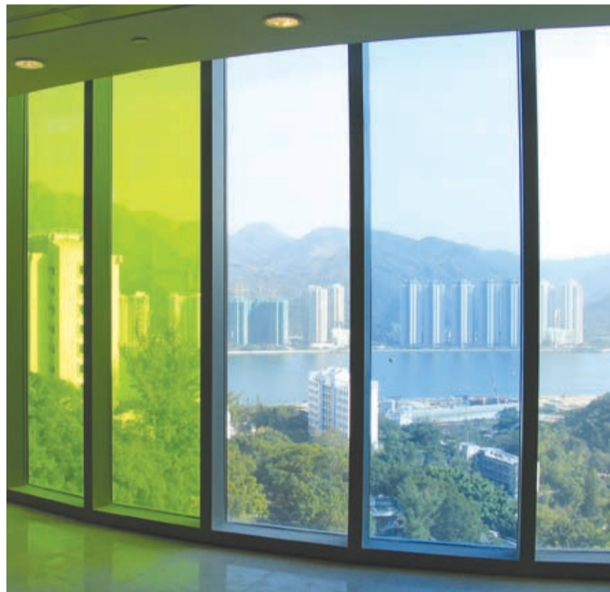
大樓正面的絕緣玻璃組件 Story-high, insulated glass units on the southern façade of the Centralized Labs
