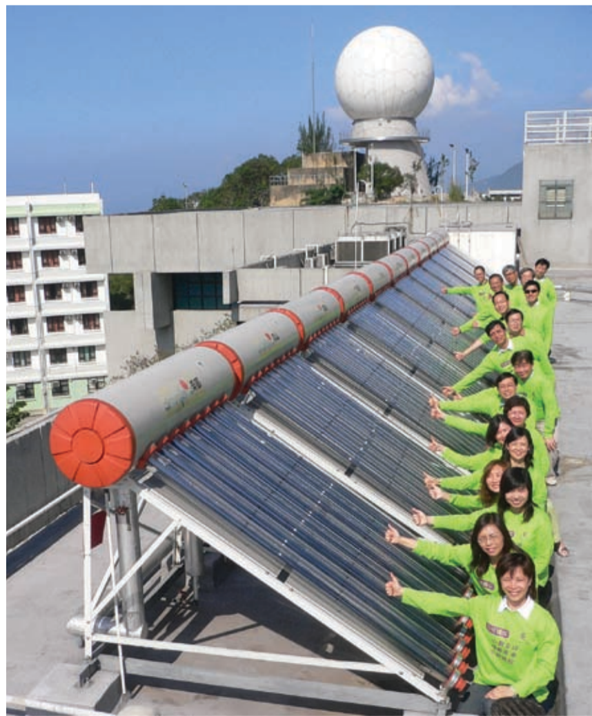
張祝珊師生康樂中心的太陽能熱水器 The solar hot water system at the Cheung Chuk Shan Amenities Building
