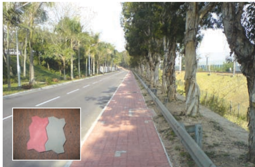
環迴東路鋪上環保地磚 Eco-glass blocks on Campus Circuit East
