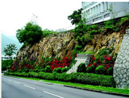
📍 Below the Tsang Shiu Tim Building, United College Simple and effective greening — two steel wires fixed horizontally on the slope act as a kind of trellis for the upward growth of bougainvillea
