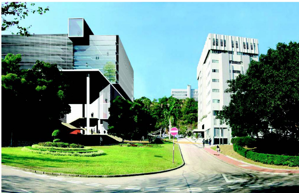
The new integrated building (left, computer rendition) to replace the Li Dak Sum Building is directly opposite to the Tin Ka Ping Building (right). In a few years, the Western campus will become a uniquely styled academic and teaching hub, one that strikes an interesting contrast with the older buildings to the east of the Tin Ka Ping Building.
