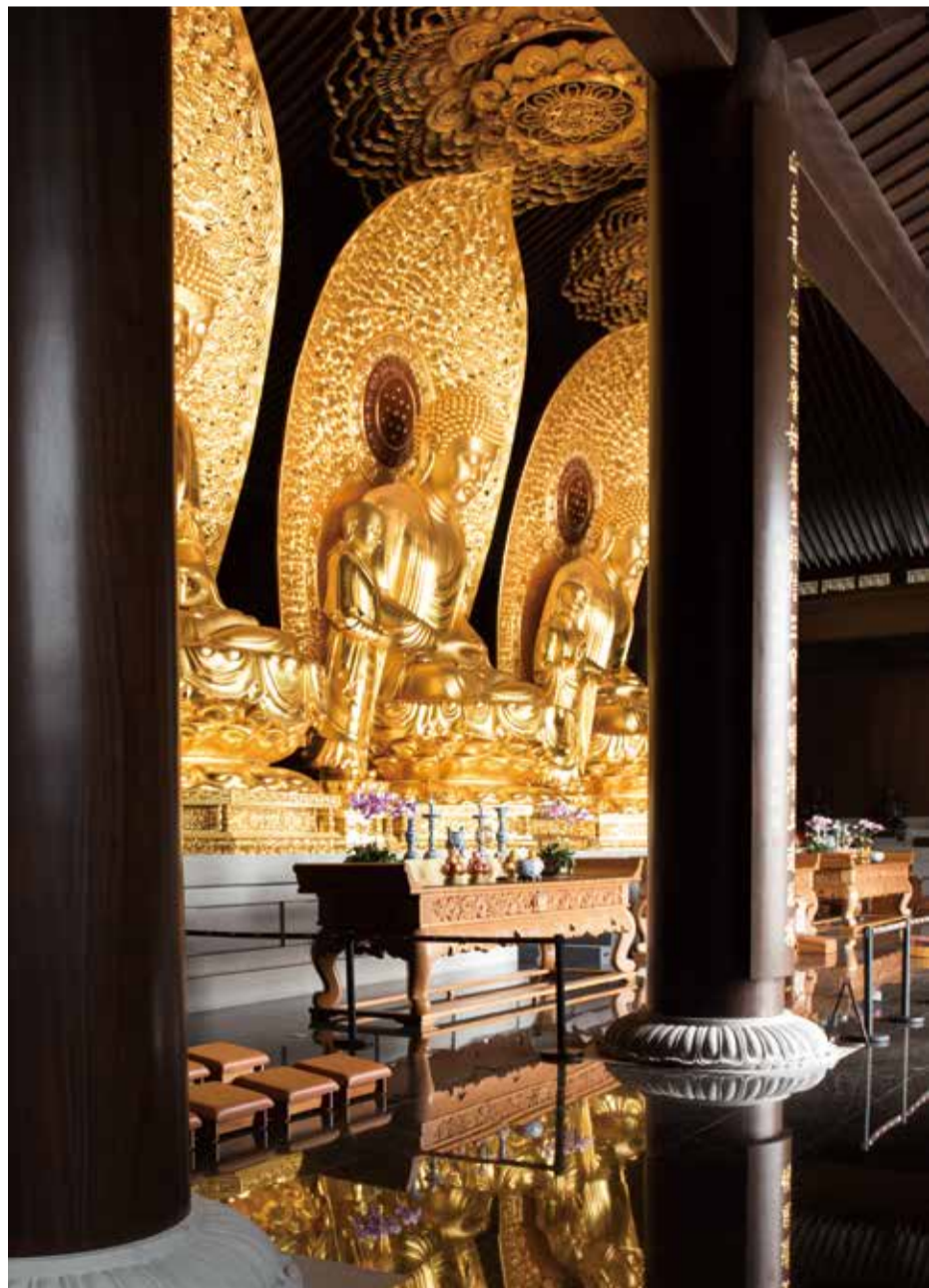
大雄寶殿的菩薩像和裝飾柱子。柱子為鋼造，柱身包以非洲紫檀木，柱座則包以石 Buddha statues and decorative pillars inside the Main Hall. The pillars are steel encased in African zitan wood and stone (base part)
