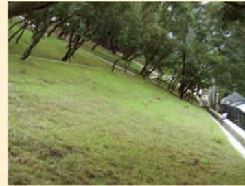
在斜坡上人工種植的樹木，是斜坡工程的一部分。這種方法可盡量減少植樹成本，但必須定期人工護理，保持樹木生長。 A more time-consuming method of stabilization—tree excavation—was used to stabilize this fill-slope near the Lady Shek Building as tree removal can be minimized. Part of the procedure was carried out manually.
