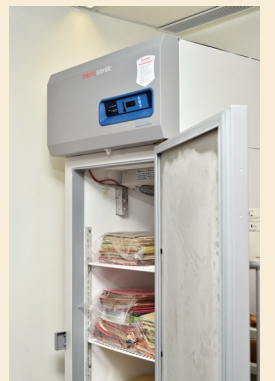
消毒文件用的冷凍櫃 The freezer for sanitizing documents
