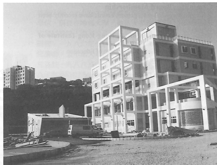
The Shanghai Fraternity Association Research Services Centre nearing completion
