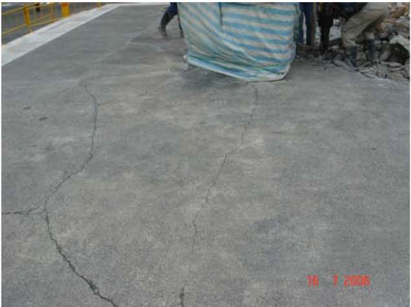
Remove damaged and sagged slab
