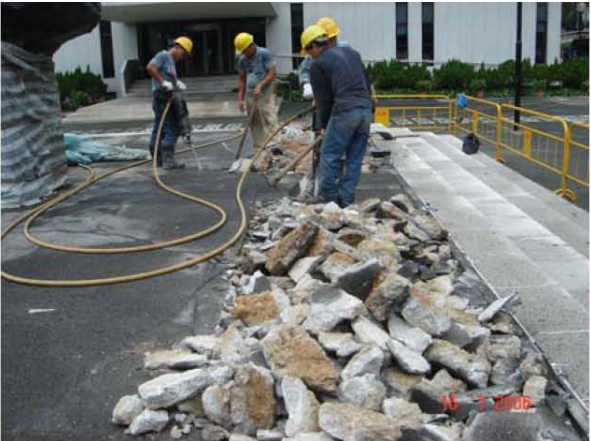
Repair surface slab at Beacon – year 2006
