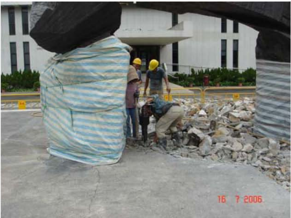
Remove damaged and sagged slab
