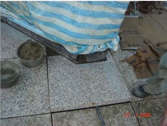
Laying 600mm x 600mm panel for slab
