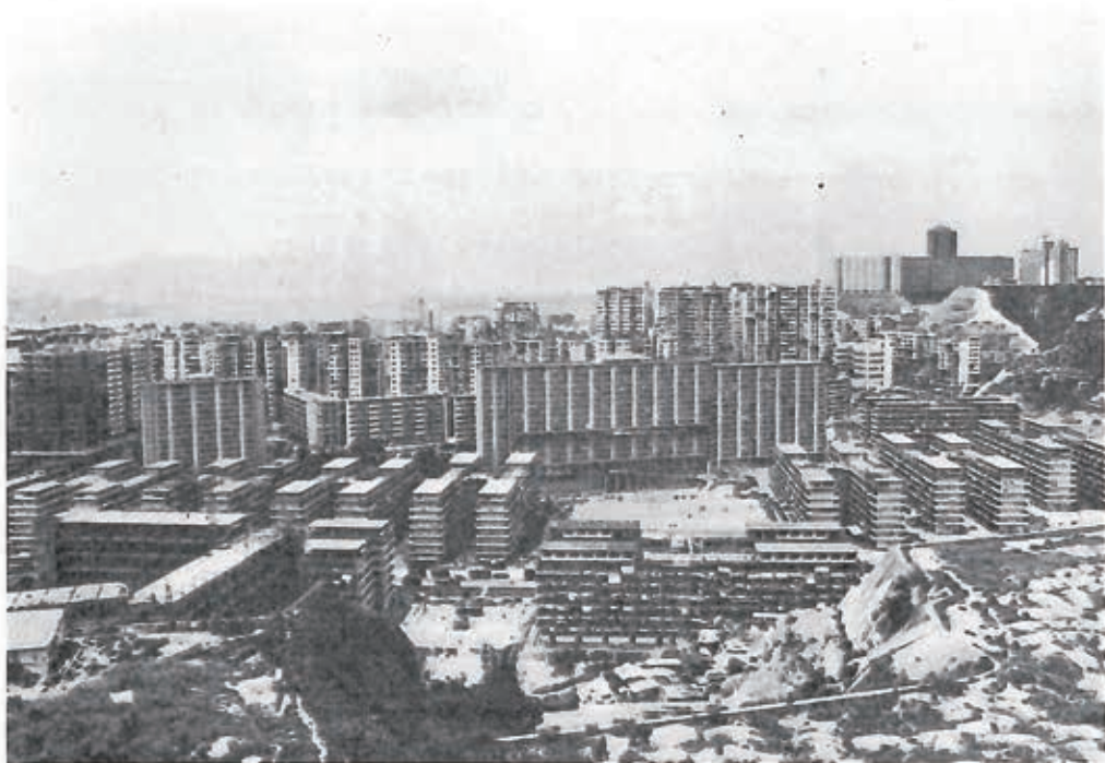
A panoramic view of the centre of Kwun Tong looking from the hills of Sau Mau Ping. The seven-storied H-shaped blocks across approximately the middle of the picture are the Kwun Tong resettlement estates (Mark I). The more modern-looking and much taller buildings behind them are low cost housing blocks of Wo Lok Estate. Further behind are multi-storied private apartment buildings.
