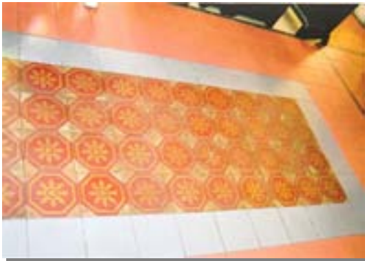
Tile mosaic found inside the Church of St. Francis Xavier, laid down in "carpet" pattern.
